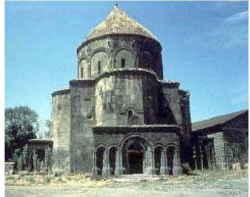
Church of Soradir, at Kars, used today as a storehouse for animal feed
