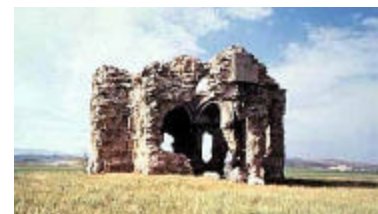
Kumbet kilise, all facing stones removed
